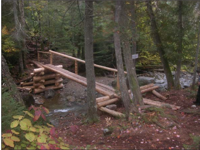
THE NEW FOOTBRIDGE OVER LILLIAN BROOK.
