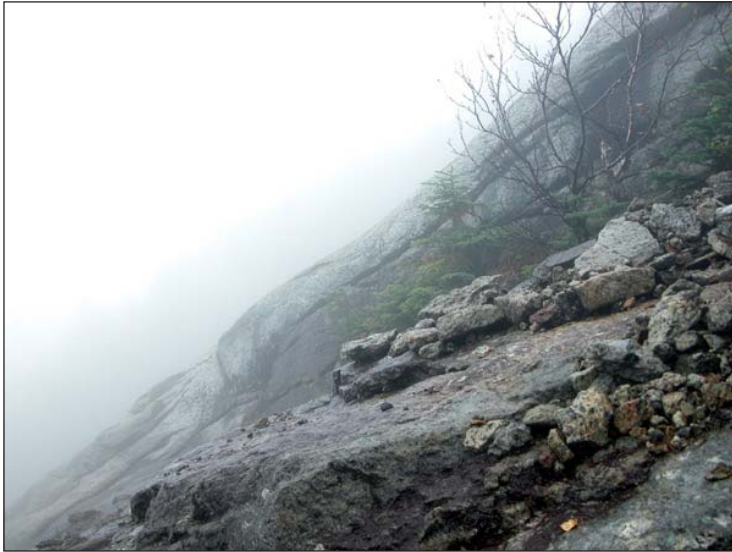
LOOKING ACROSS THE SLIDE, THE GRADE IS EVIDENT DURING A PARTICULARLY STEEP SECTION
